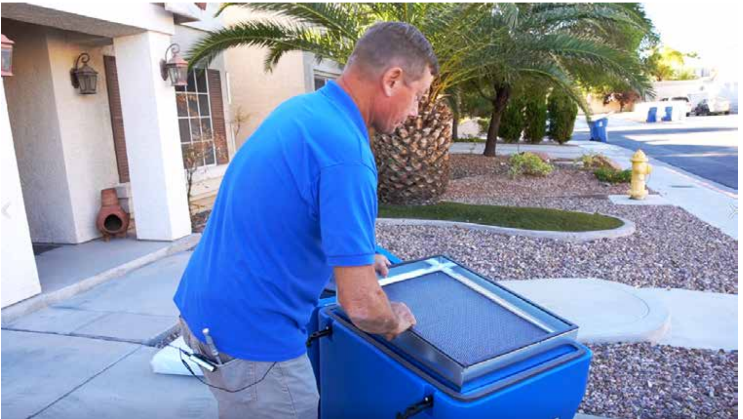
Third Stage HEPA Filter
