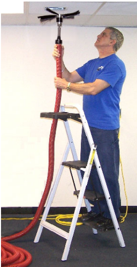
Cleaning Ceiling Ducts
