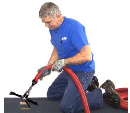
Cleaning Floor Ducts
